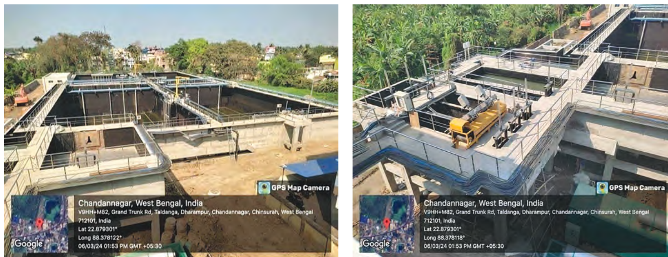
Figure 139 STP at Hooghly-Chinsurah Municipal Area
