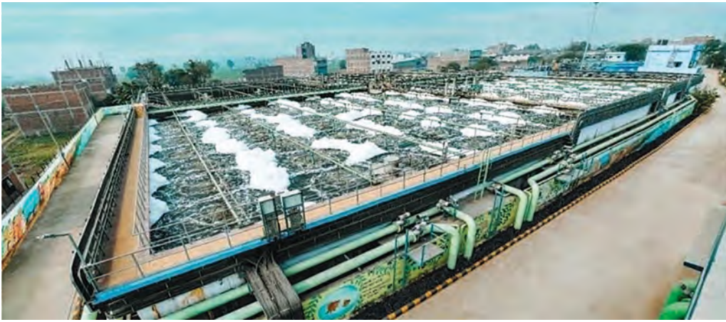
Figure 128 Karmalichak STP Network 37 MLD
