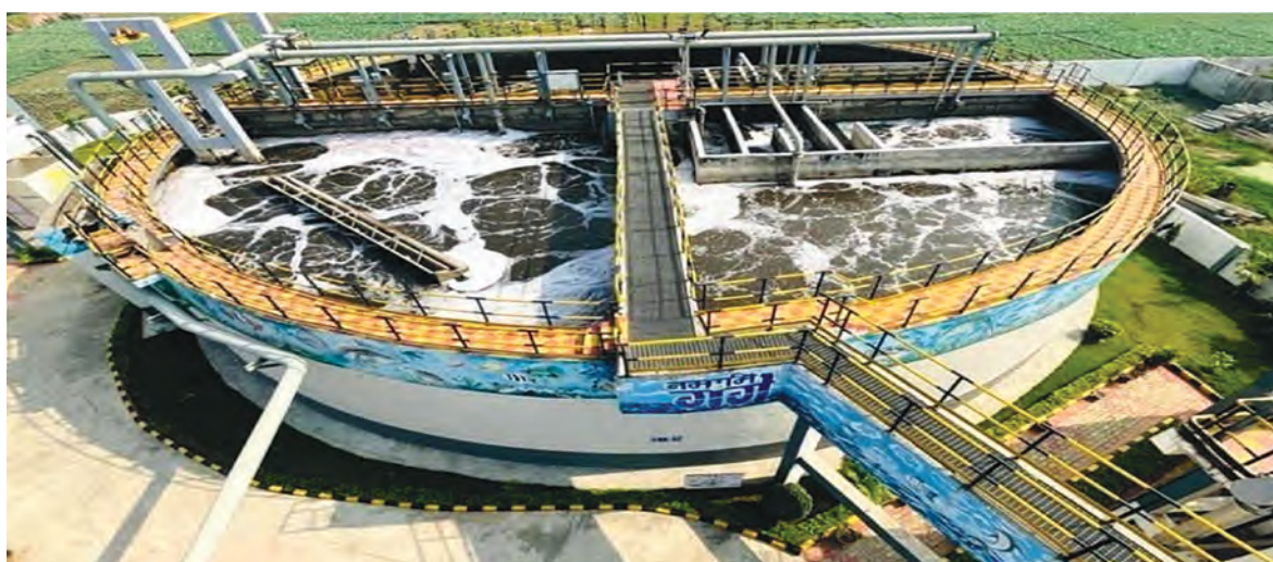
Figure 132 Barh STP and I&D work 11MLD
