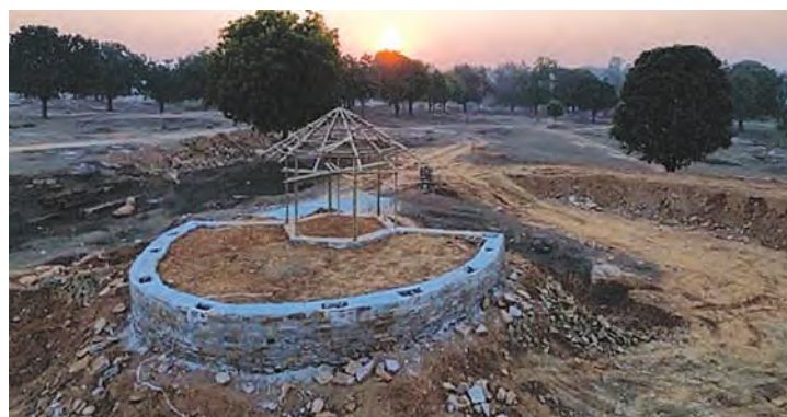
Round Hut Construction
