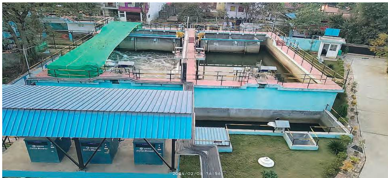
Figure 134 Sonepur STP and I&D work 3.5 MLD
