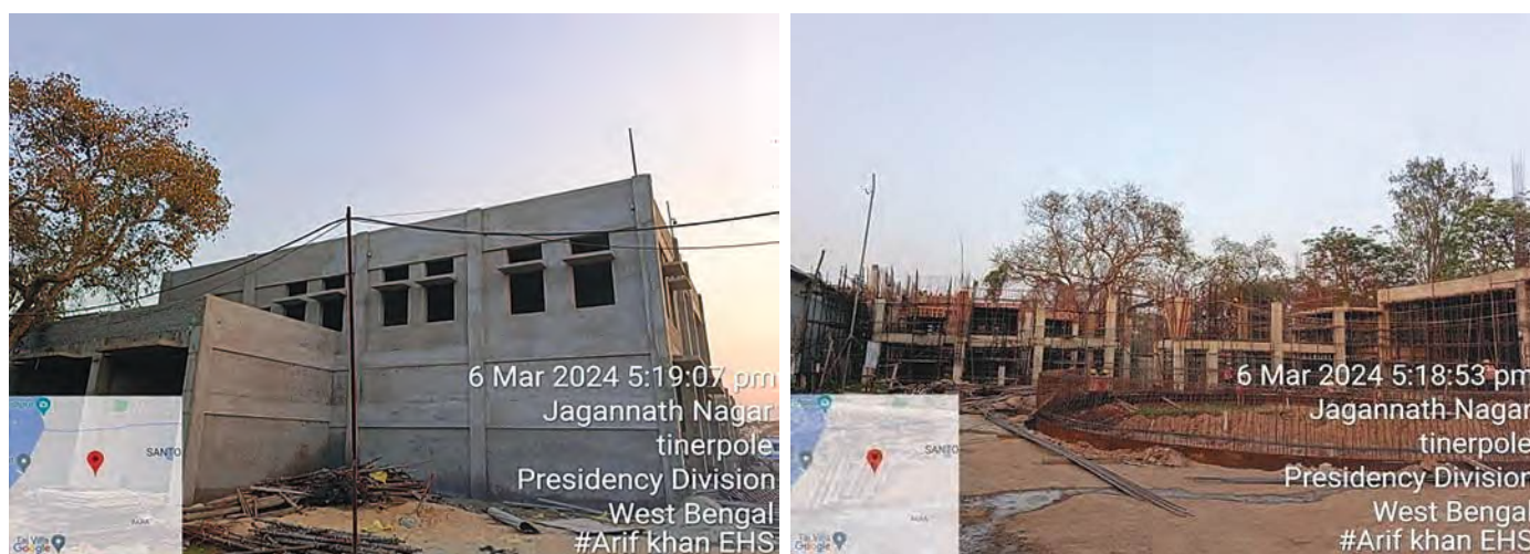
Figure 140 STP at Maheshtala Municipality
