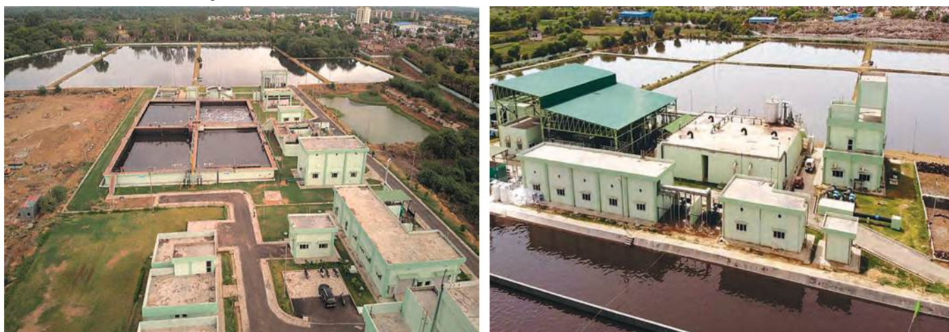
Figure 109 Tertiary Treatment Plant, Mathura
