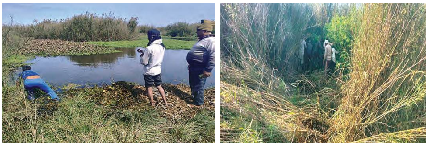
Kalewala Jheel Wetland, Muzaffarnagar: Site cleaning & clearing weeds
