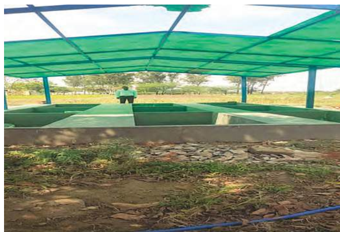
Developing vermi-compost facility
