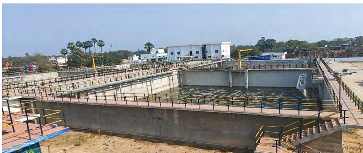
Figure 135 Chhapra STP and I&D work 32 MLD
