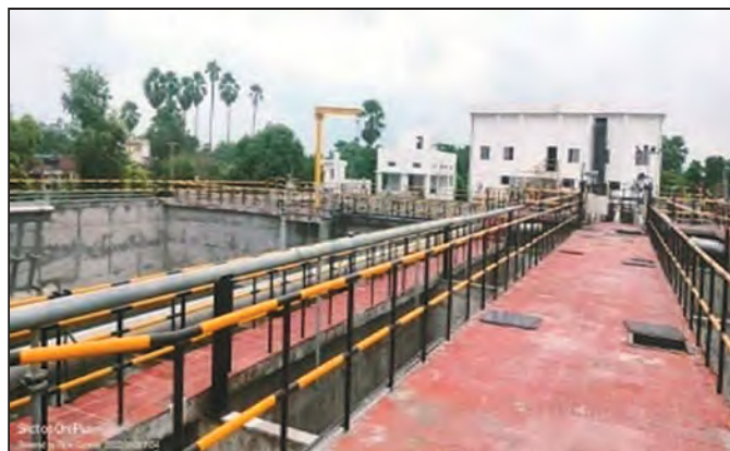
32 MLD STP at Chhapra
