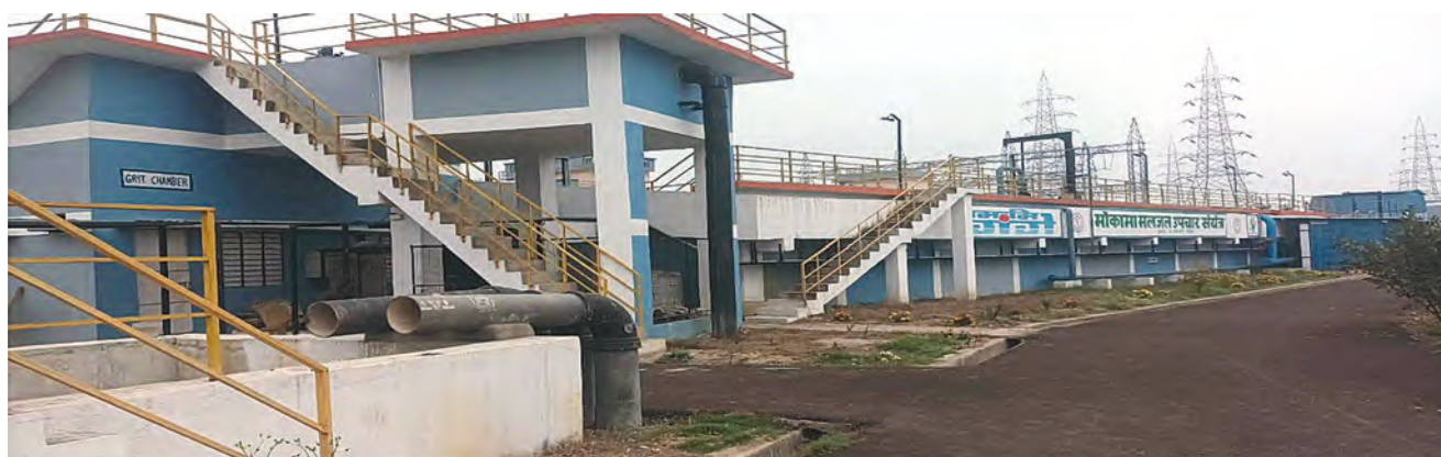
Figure 133 Mokama STP and I&D work 11MLD
