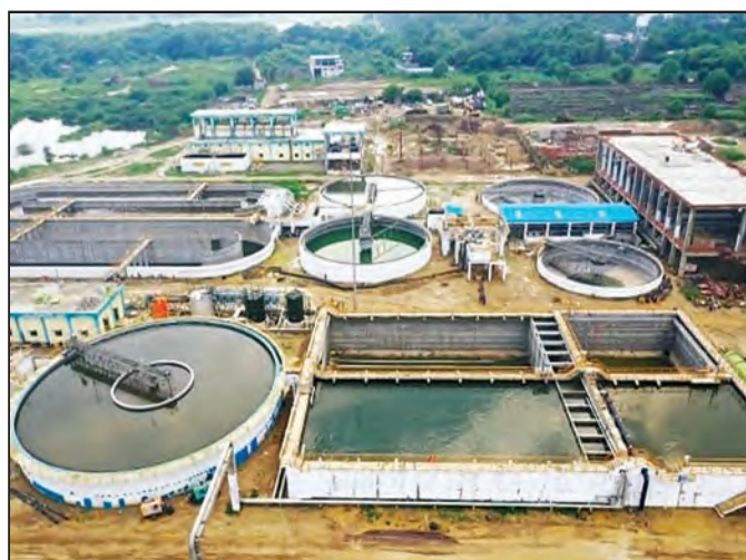
20 MLD CETP for Tannery Cluster at Jajmau
