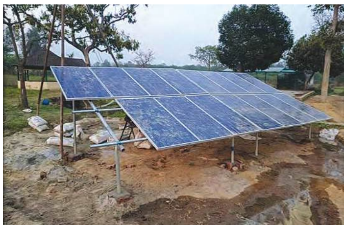
Solar pump installation
